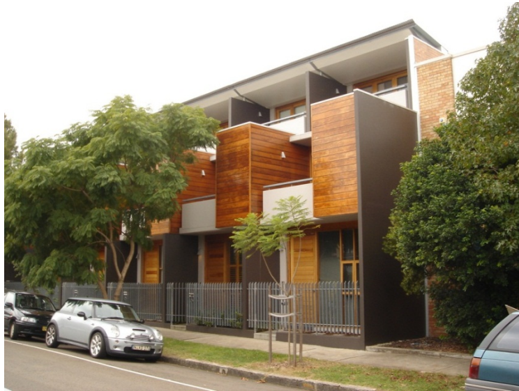
Figure 5.x: Terrace houses in Lawrence Street, Alexandria
